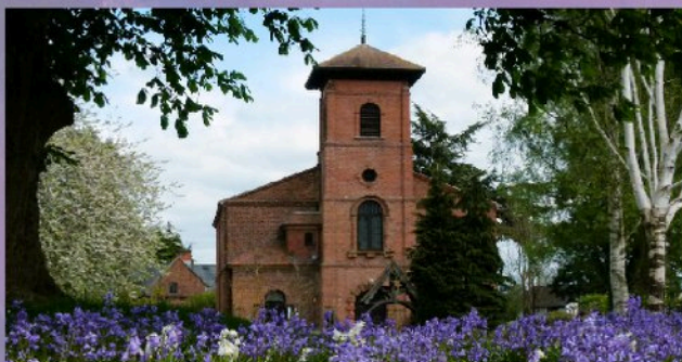
Whittington Church, Shropshire SY11 4DF
